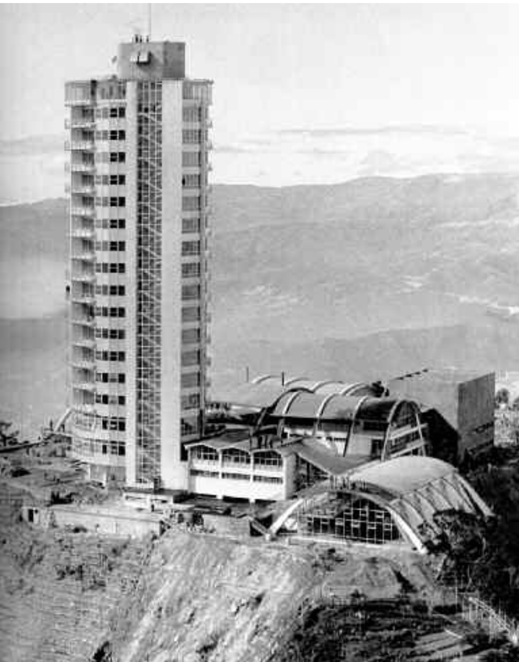
Figure 4 Hotel Humboldt (Tomás Sanabria, 1955). AFU
