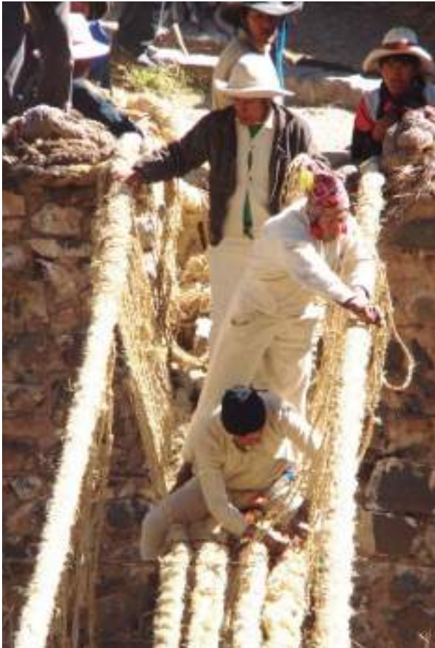
Third day. The Chakaruwaq usually finish the construction of the bridge around mid-afternoon. Source: Roel et al. 2015, 173.
